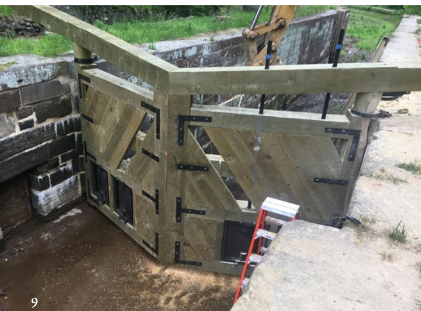
7 Tuning the miter joint between the two gates.
