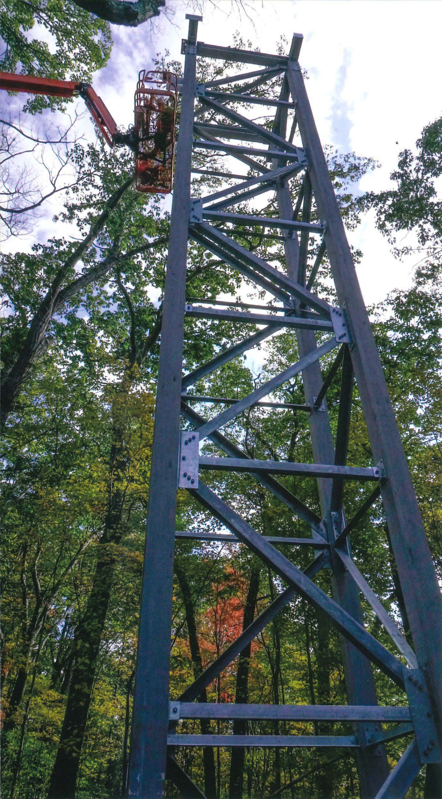
8 A braced frame tower along the stretch of walkway connecting the Tree House to the proposed terminus building—column glulams each over 50 ft. long. With post base assemblies and concrete piers, the deck of this tower was almost 60 ft. above the forest floor.
