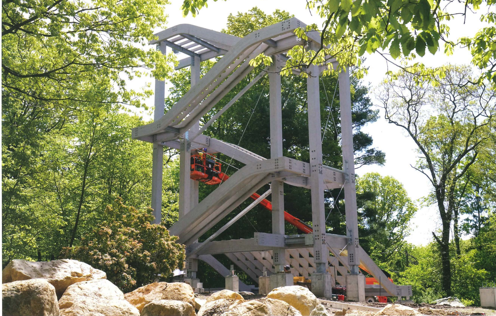
9 The fully erected Tree House, midway along the walkway. Built-up bleacher and stair stringers installed. There is a large set of bleachers at the lower level and another, smaller set at the top. The main glulam columns here are 16x16, up to 45 ft. long.
