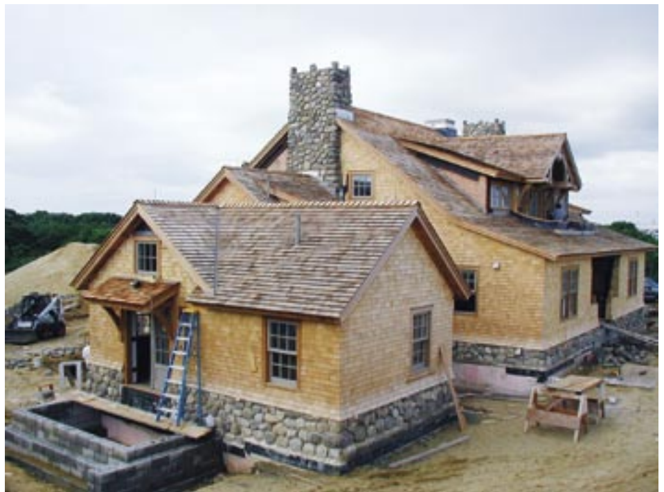
Nantucket residence, view of exterior near completion. General contractor: Woodmeister Corp.
