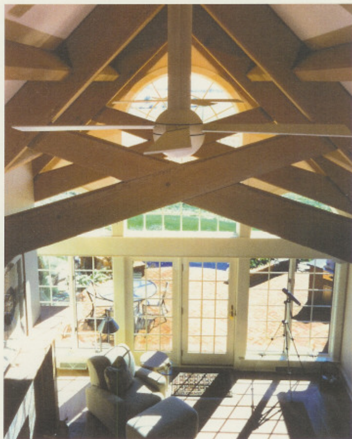
This scissor truss conveys a timber-frame look in a conventionally framed house.
