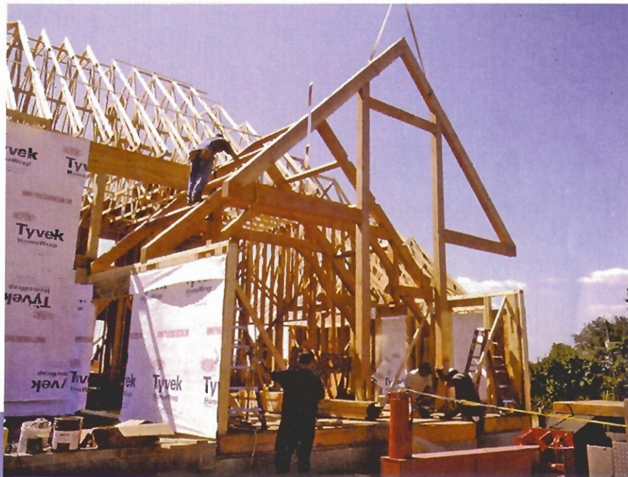
Here, with the assistance of the crane, the gable truss is held in position while the tenoned purlins are dropped into place, stabilizing the roof structure.
