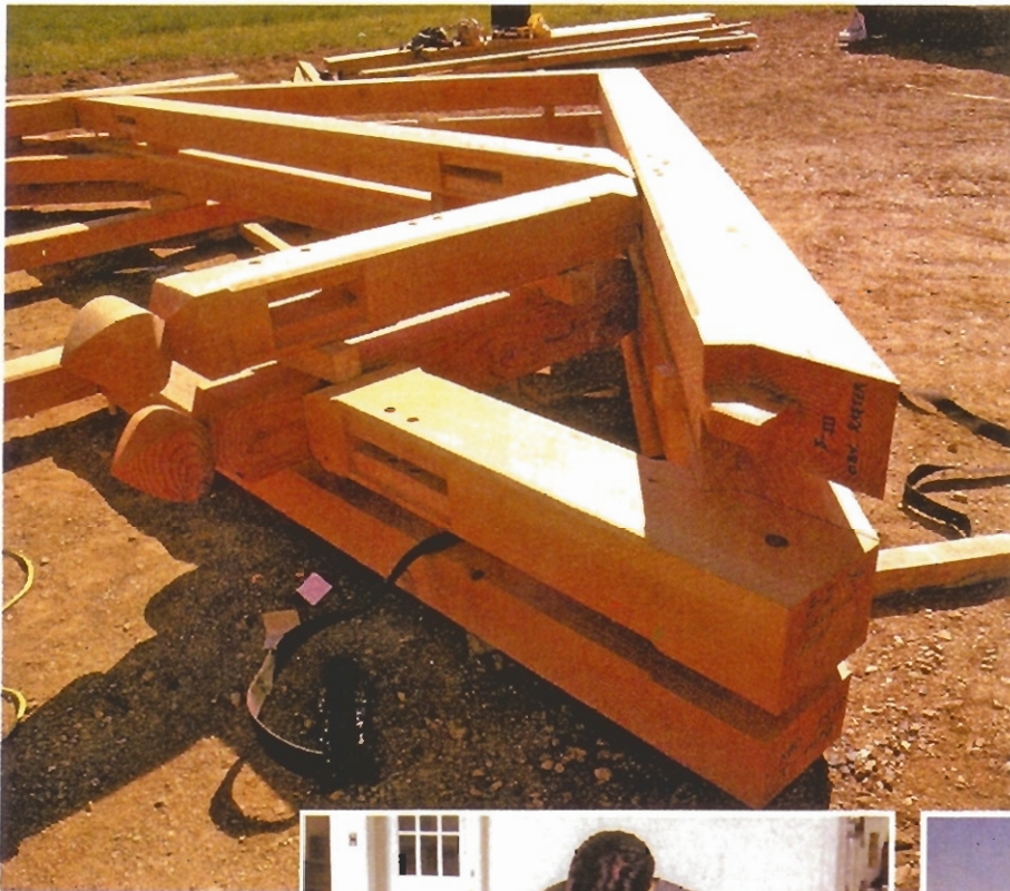
Trusses are prefabricated and bored in the shop (below left), then reassembled on site in preparation for lifting with the crane (below).
