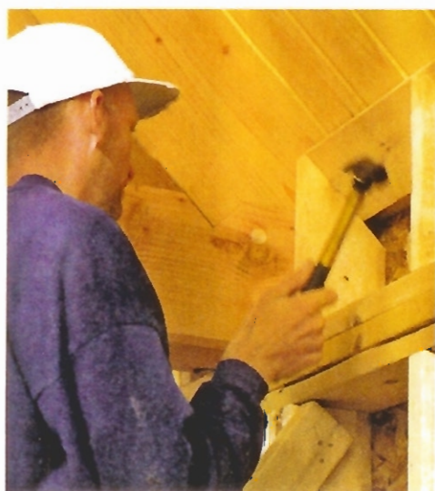
Working on the "no nail zone," a carpenter prepares the knee-brace mortise in a 2x6 support post (above). The knee brace is then persuaded into place (above right). On this job, the top-sloped "mini wall" was added after the trusses (right).
