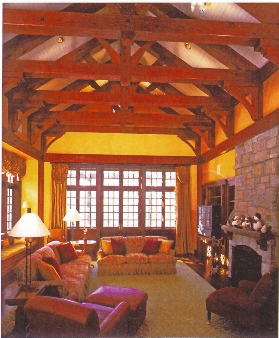
Depending on the details, timber trusses can evoke a traditional — even medieval — feeling or fit nicely in a contemporary space. At left are strutted king-post trusses with bracketed knee braces underneath; below, scissors trusses with horizontal purlins.
