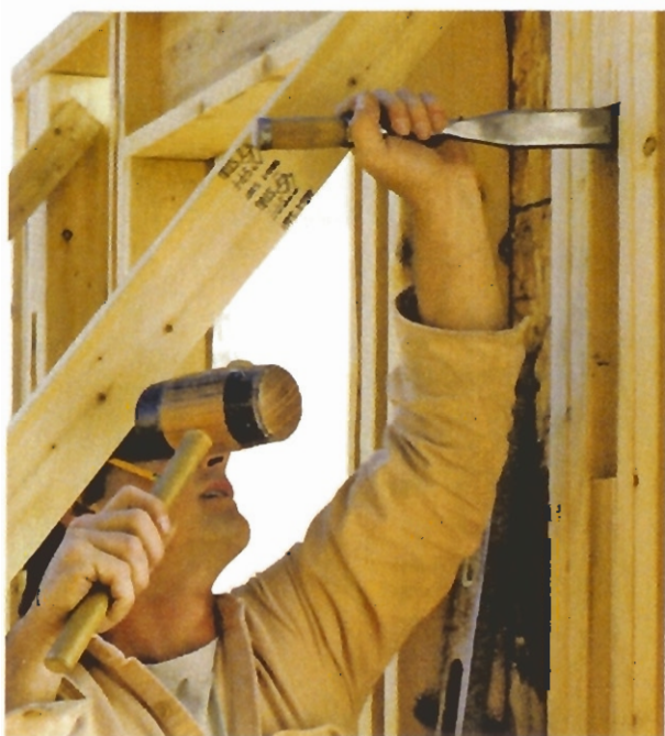
Working on the "no nail zone," a carpenter prepares the knee-brace mortise in a 2x6 support post (above). The knee brace is then persuaded into place (above right). On this job, the top-sloped "mini wall" was added after the trusses (right).
