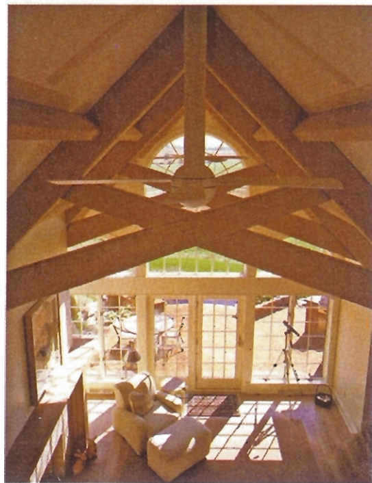
Depending on the details, timber trusses can evoke a traditional — even medieval — feeling or fit nicely in a contemporary space. At left are strutted king-post trusses with bracketed knee braces underneath; below, scissors trusses with horizontal purlins.
