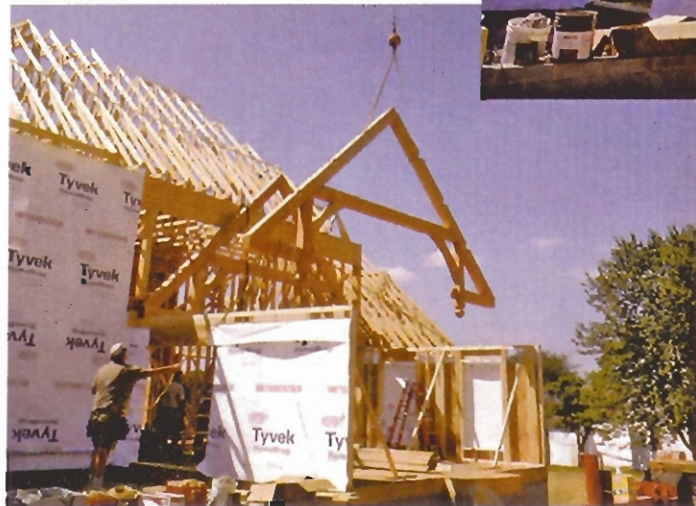
Here, with the assistance of the crane, the gable truss is held in position while the tenoned purlins are dropped into place, stabilizing the roof structure.
