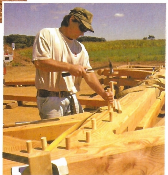
Trusses are prefabricated and bored in the shop (below left), then reassembled on site in preparation for lifting with the crane (below).
